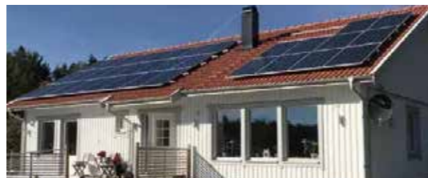
Residential Project in Sweden 10kW
