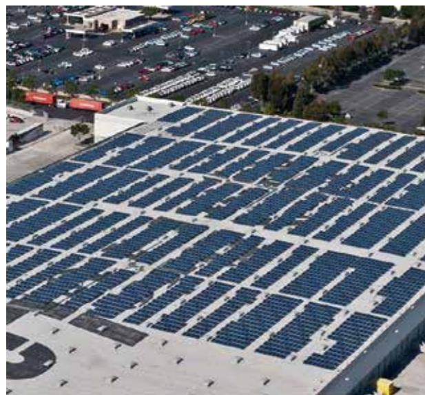
Commercial Project in Estonia 63.6kW
