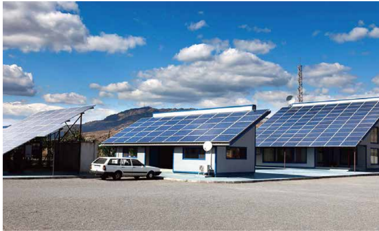
Residential Project in Indonesia 6kW
